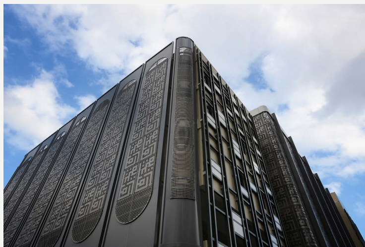
▲ The new Madrasah Al-Arabiah Al-Islamiah campus is equipped with up-to-date facilities to support the school specialisation in science-based curriculum.
