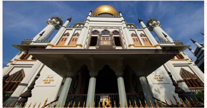
Completion of upgrading and restoration works at Sultan Mosque, 16 Jan 2016
